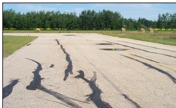
Beaverlodge Airport-Taxiway Alpha
