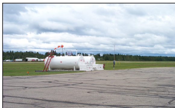
Edson Airport – Main Apron
