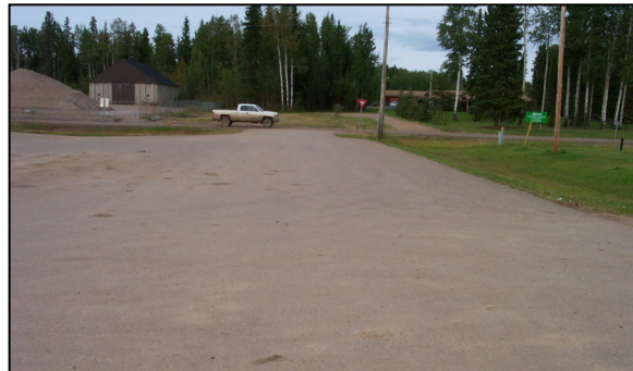
Rainbow Lake Airport – Parking Lot and Entrance Road
