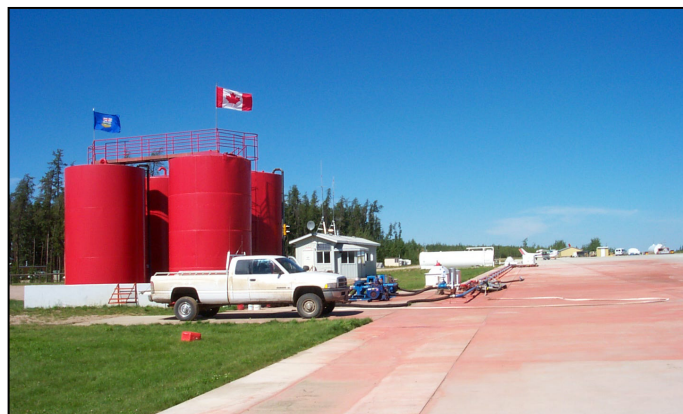
Loon River Airport –Retardant Tanks and Apron
