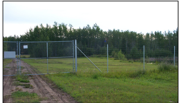
High Level Airport – Perimeter Fencing
