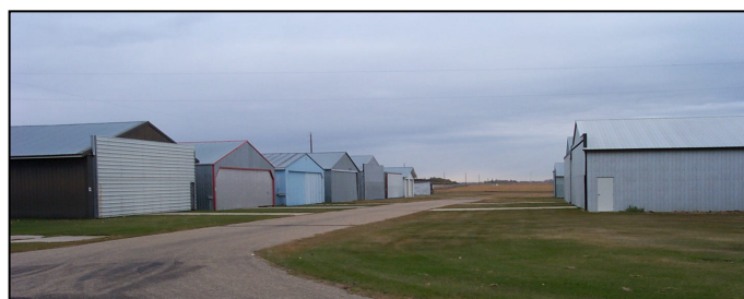
Hangars at Lacombe Airport
