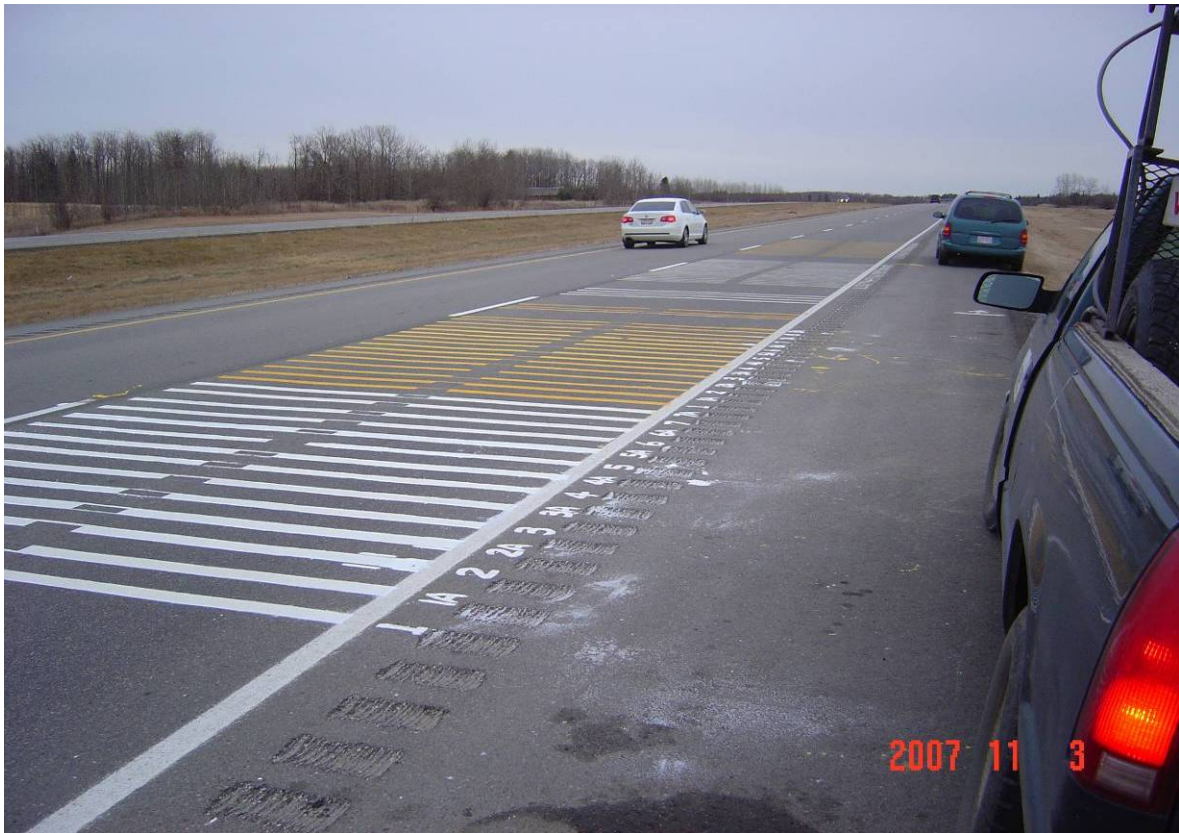
Completed application of cold temperature traffic paints (white and yellow)
