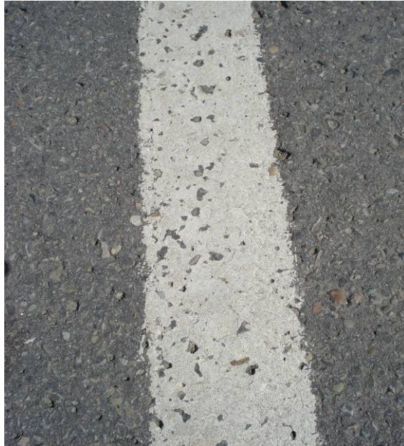
Close-up: some chipping, durability is good
