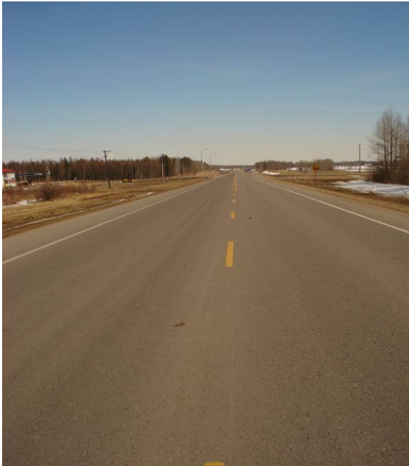
Centerline skip looking east
