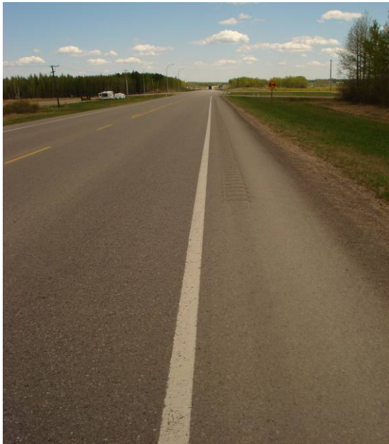
South edge line looking east
