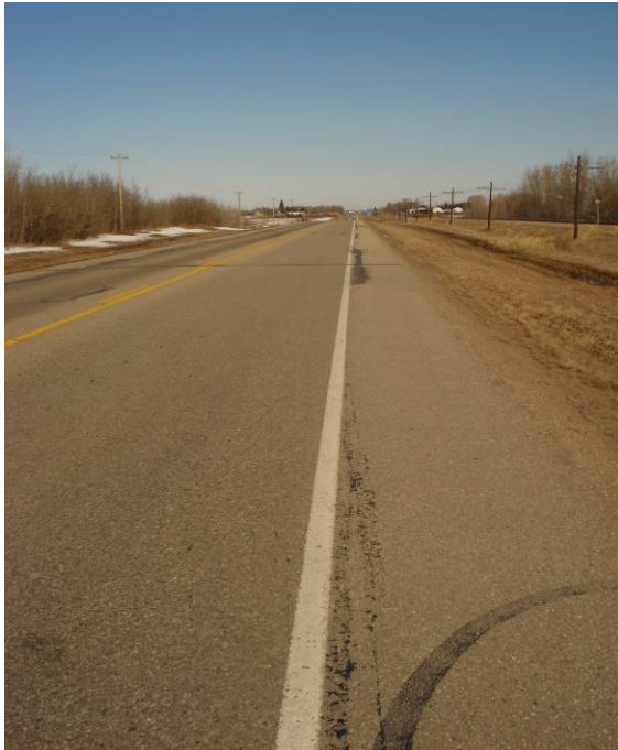
East edge line looking north
