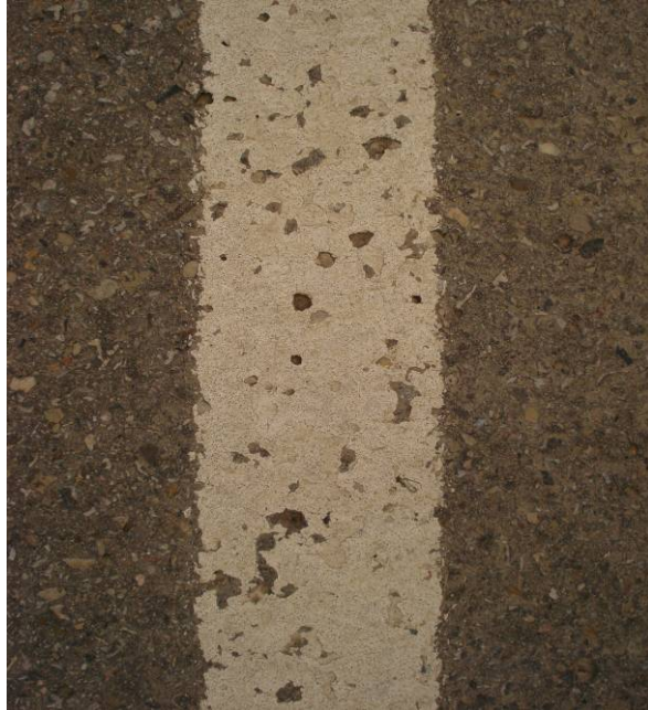
Close-up: some chipping, durability is good
