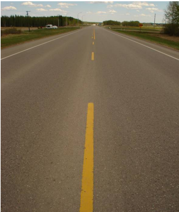
Centerline skip looking east
