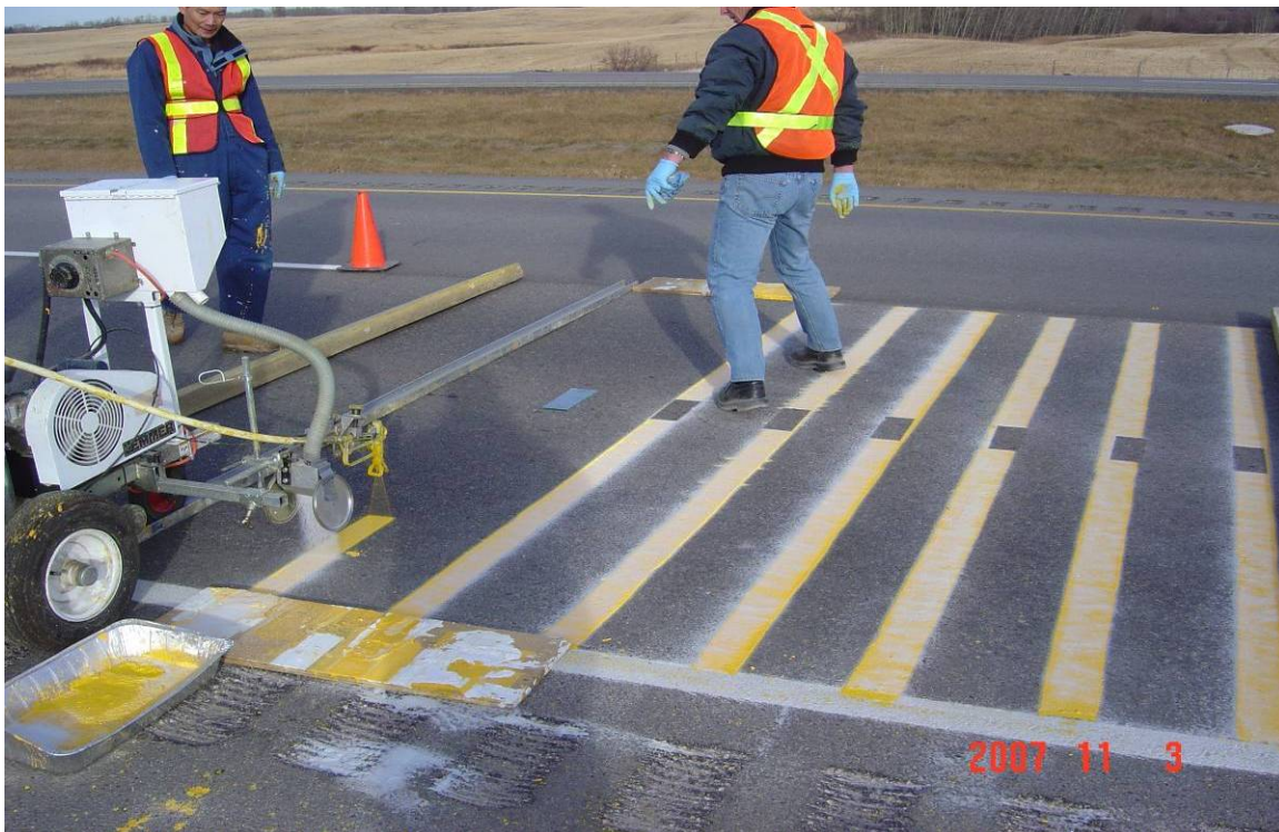
Application of paint and glass beads
