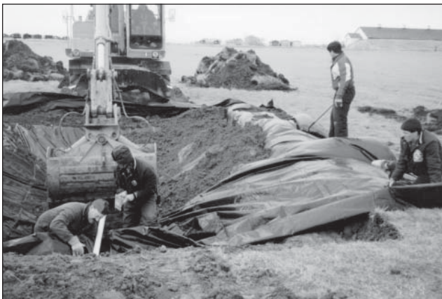
Figure 2. Installing and backfilling plastic liner
