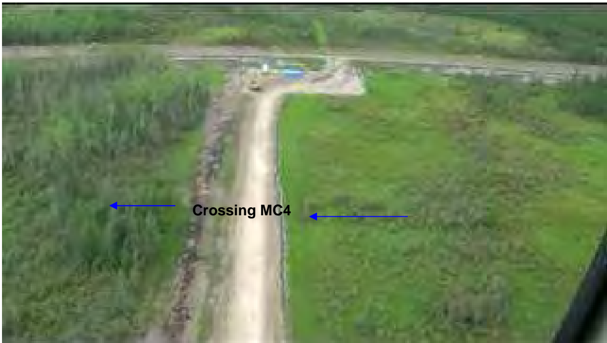
Photo 24 Drainage 6 looking north at crossing site MC4
