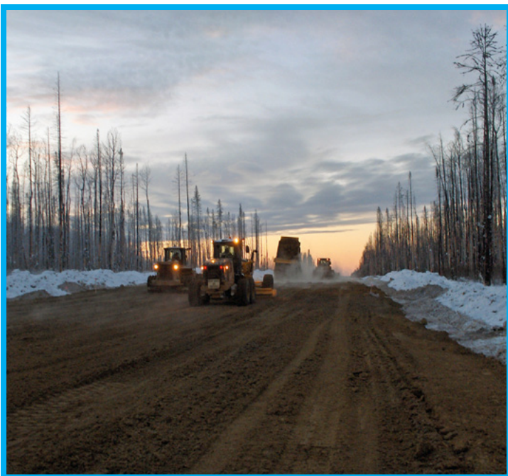
Construction on Southern Pacific's all-season access road. (December, 2010)
