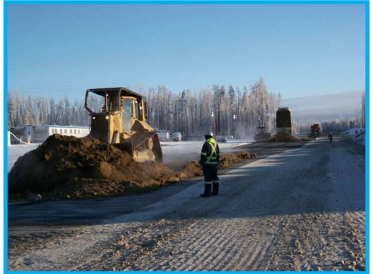
Construction on Southern Pacific's all-season access road. (January, 2011)
