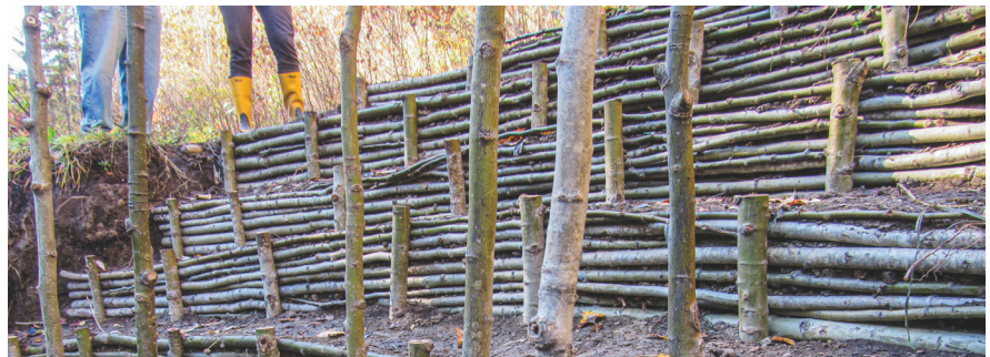
Photo by Associated Engineering
