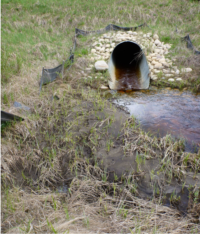
Figure 8: Slumping Example (Photo courtesy of D.Park)
