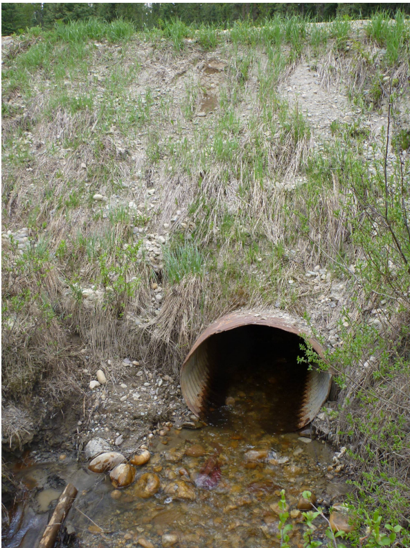
Figure 8: Slumping Example (Photo courtesy of D.Park)
