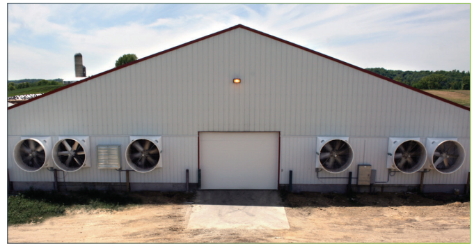
Figure 3. Mechanical Ventilation on Livestock Barn Source: www.jdmfg.com
