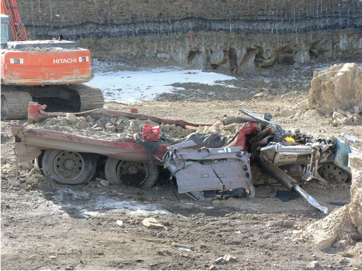
Photograph 4: Shows excavator and damaged dump truck
