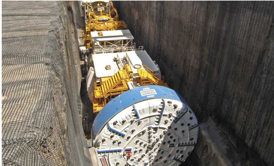
TBM LAUNCH BOX FOR THE NIAGARA HYDROELECTRIC PROJECT IN ONTARIO
