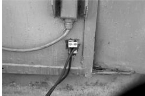
**Note double metal-to-metal connection**Equipotential bonding conductor requirements
