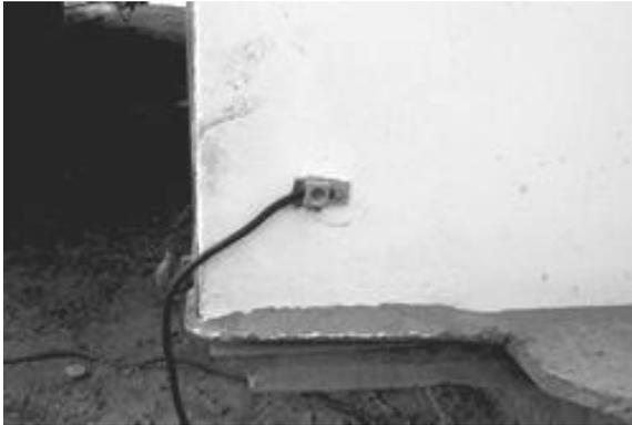
**Note single metal-to-metal connection**
