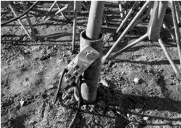
a) The rig guyline anchor (usually the closest one to the rig generator)
