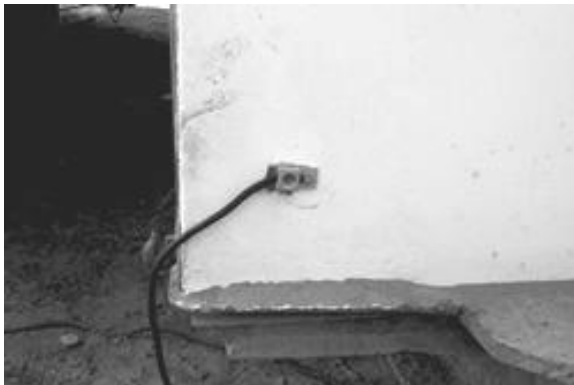
Note single metal-to-metal connection
