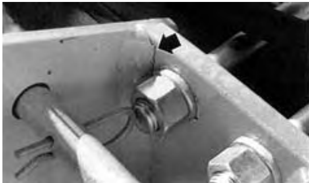
FIGURE 8. Shank Assembly Weld Cracks.
