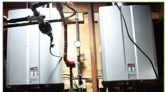
Figure 5. Tankless Hot Water Heaters
