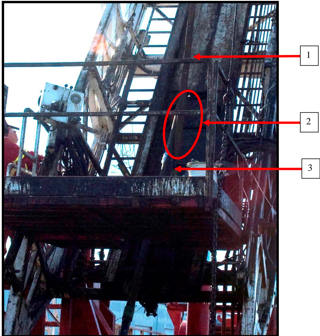
Photograph 9 – Shows a re-creation of the incident site.
