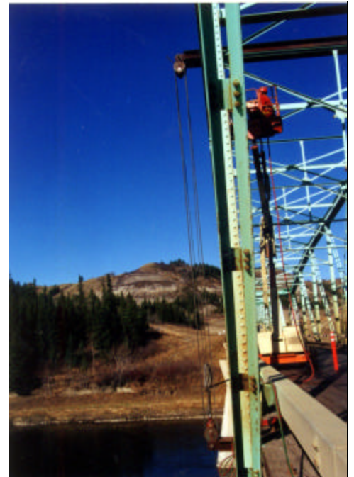
A truss tie may be required if repairs are needed for severely damaged tension members.
