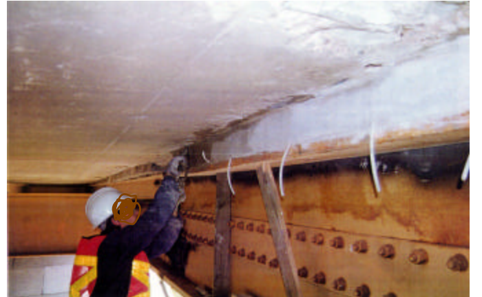
...loose concrete is removed, the haunch patched and the crack is epoxy resin injected. Installing injection ports.
