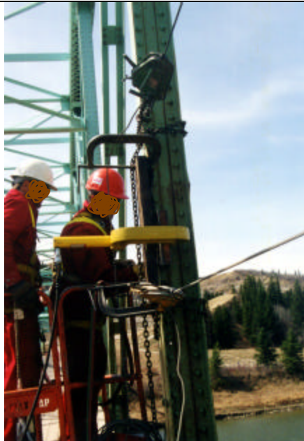
Effective heat straightening procedures may require several combinations of external force application with various heating patterns and techniques.
