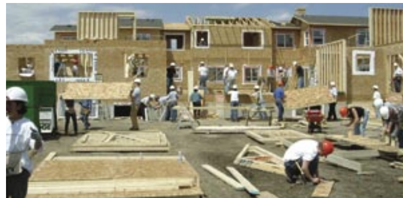
Habitat for Humanity framing day for TransCanada June 26, 2004
