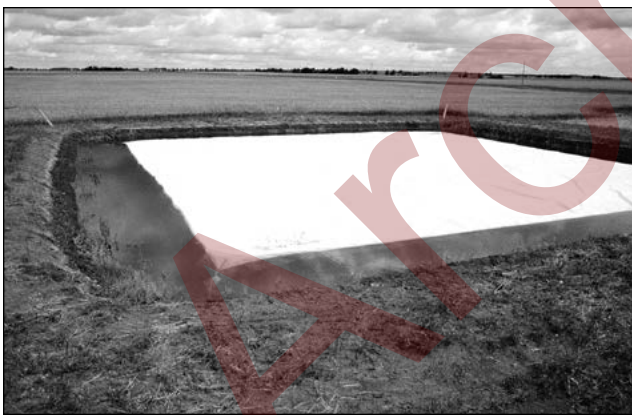
Figure 4. Plastic cover to reduce dugout evaporation losses
