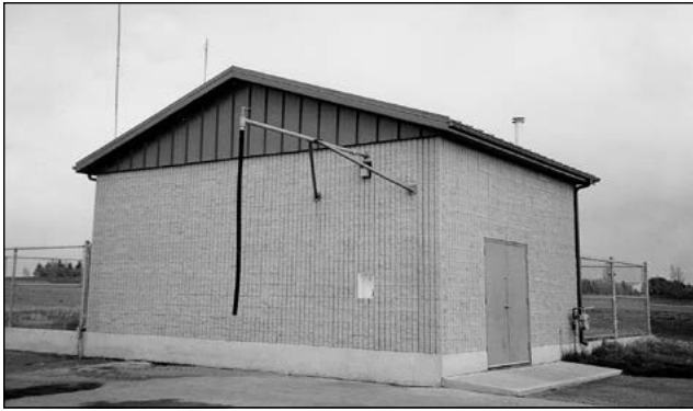
Figure 5. Tank loading facilities
