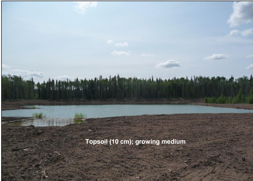
Figure 5.0 Constructed Wetland Features Placement of topsoil; growing medium
