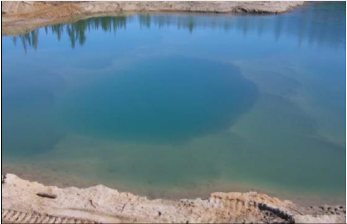
Figure 3.0 Constructed Wetland Features Deep hole located at the north end of the constructed wetland
