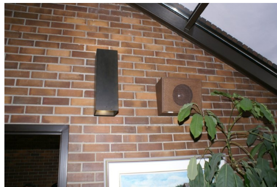
Existing main stairwell lighting
