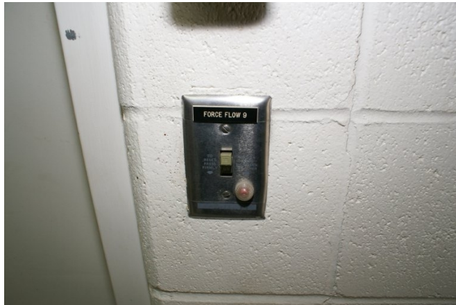
Manual motor starter c/w pilot light
