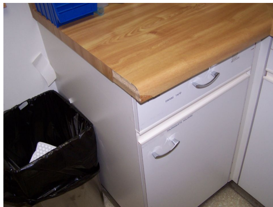
Laminate missing for counter top
