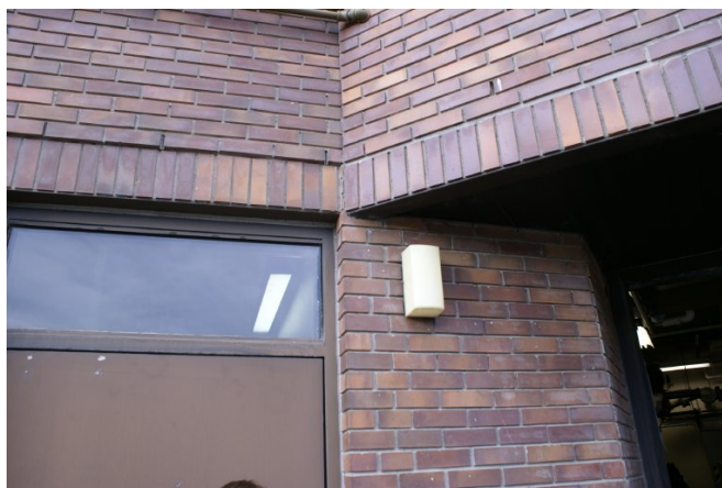
Incandescent wall mounted fixture.
