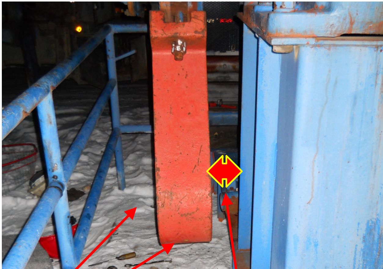
1 2 3 Side view of pump jack counterweights showing crushing location.
