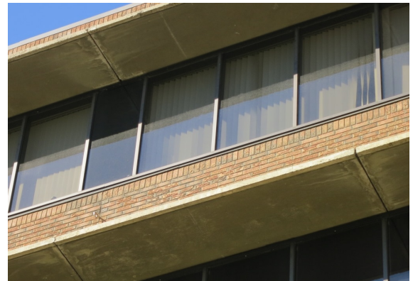
Concrete sun shades on south elevation.
