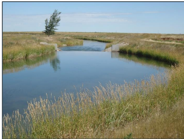
Inflow to Fincastle Reservoir in the Taber Irrigation District
