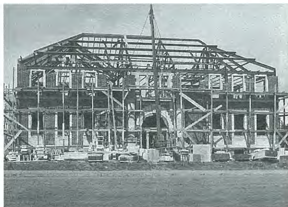
Court House under construction, 1930.
