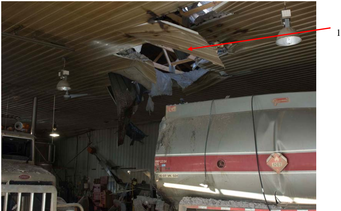
Photograph 6 – Shows the damaged highway transport vessel following the explosion in the building. The picture was taken through a window opening.
