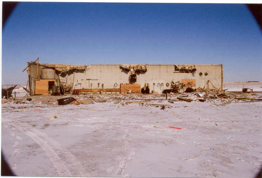
Photograph 7 - Shows the building following demolition.
