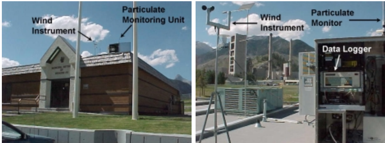
Figure 2.1 Particulate and wind instrumentation on top of Municipal District of Bighorn #8 building in Exshaw.
