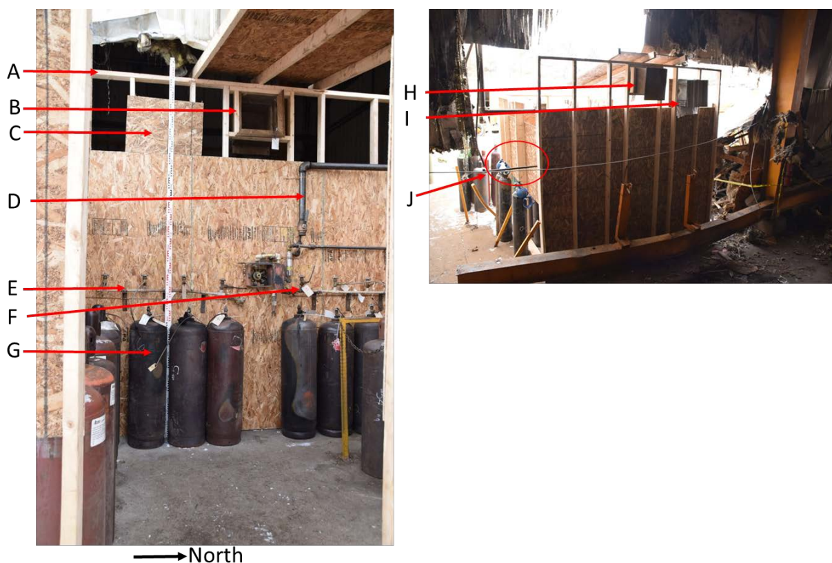
Figure 6. Re-constructed Exemplar acetylene storage shack, front view and rear view. The manifold system provided continuous acetylene to Shop 1.
