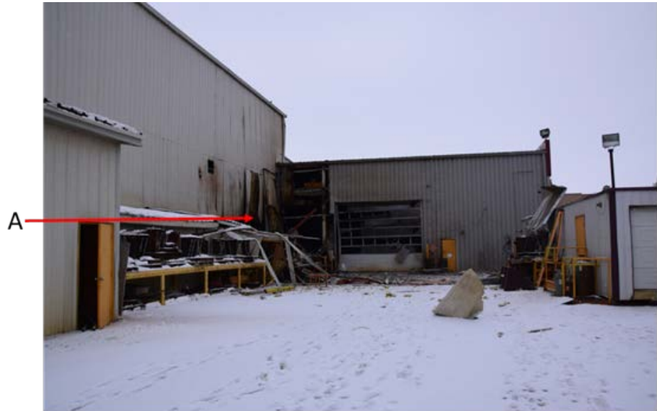
Figure 14. Acetylene shack post explosion facing north long shot of the incident location from outside Bay 9.
