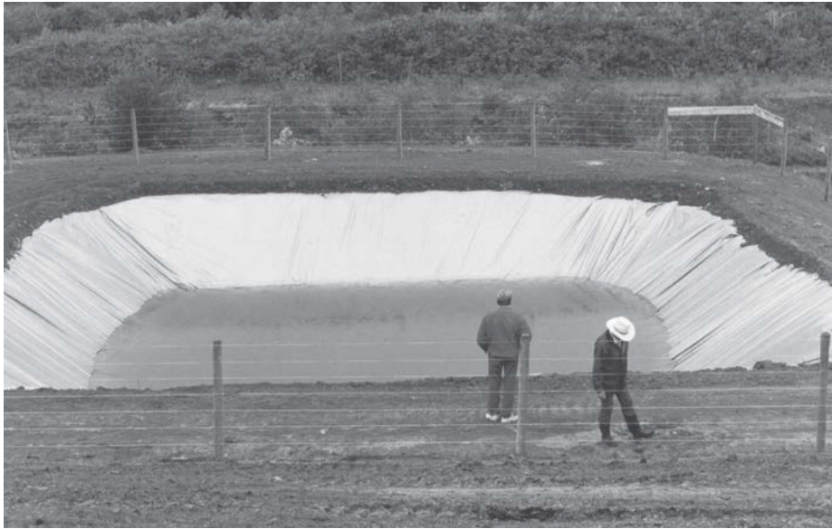
Figure 5-12 Elevated Earthen Reservoir with Woven Polyethylene Liner
