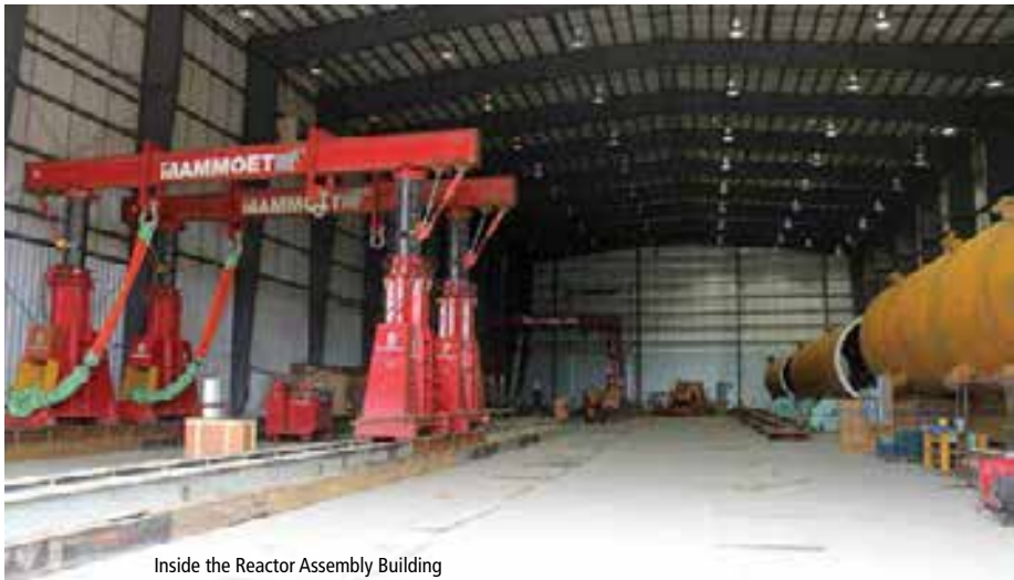
Inside the Reactor Assembly Building
