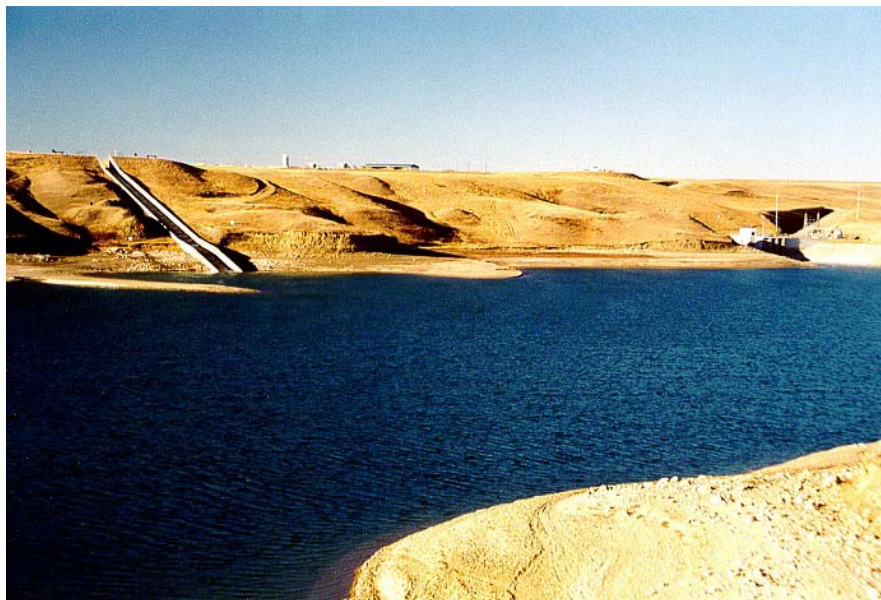
Figure 4.10: Chin Reservoir South of Taber
