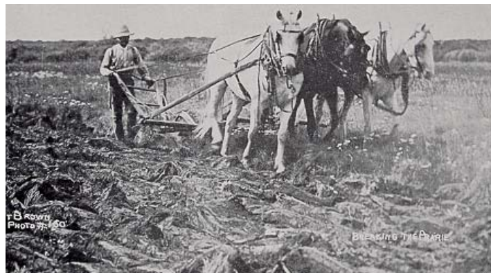
Figure A.16: Breaking the Sod
