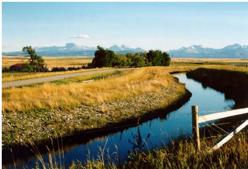
Figure 4.14: Surface Distribution Canal
