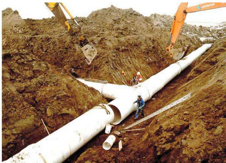
Figure A.5: Buried Pipeline Installation
