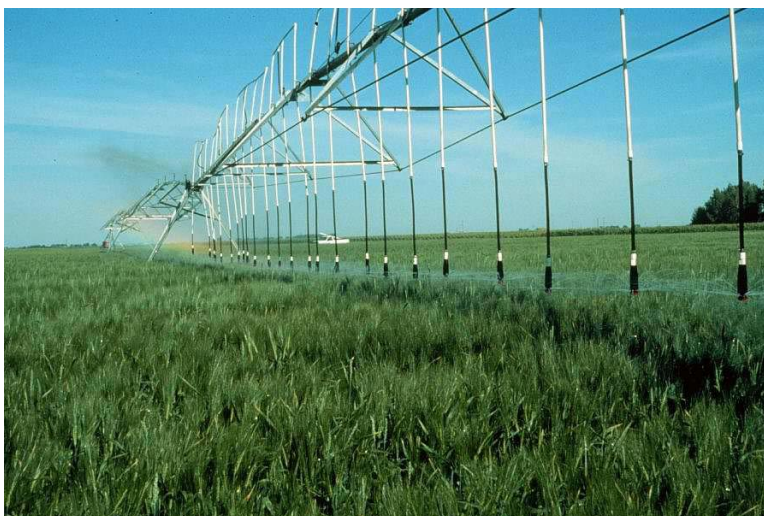
Figure A.7: Drop-tube Low-pressure Irrigation Pivot
