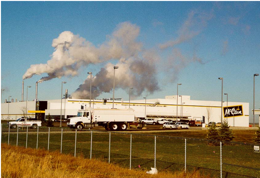
Figure A.22: Potato Processing Plant East of Lethbridge
