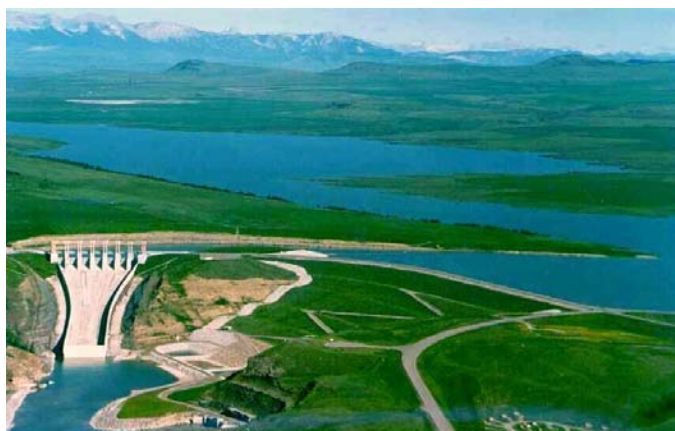
Figure A.2: Oldman Dam and Reservoir
