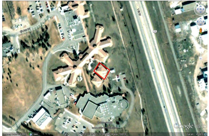
General view of the Site.
