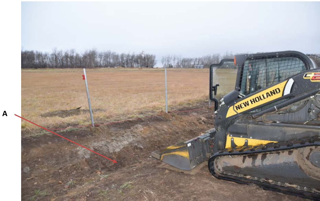
Figure 3. Perspective facing northwest indicating the fence posts running north – south. The depression running parallel along the east side of the fence indicates non-level terrain.
