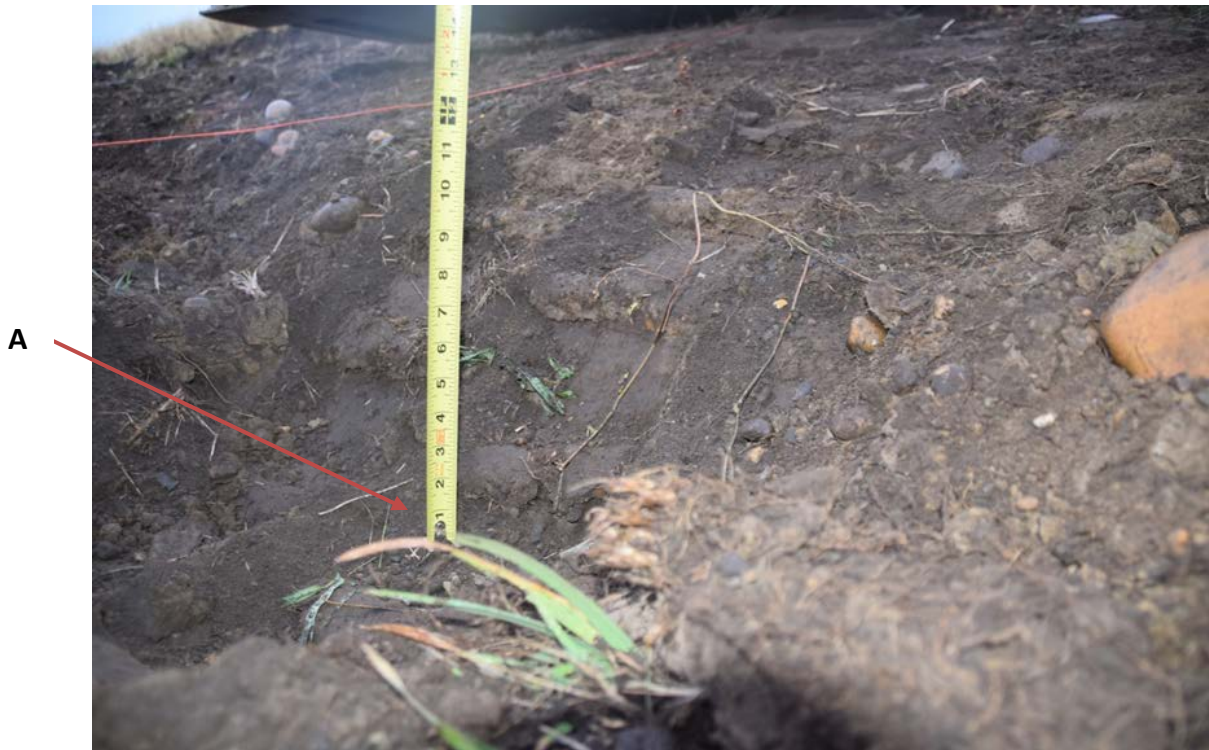
Figure 5. The depth of the depression, measured post-incident, was approximately 30.48 cm (12 inches).
