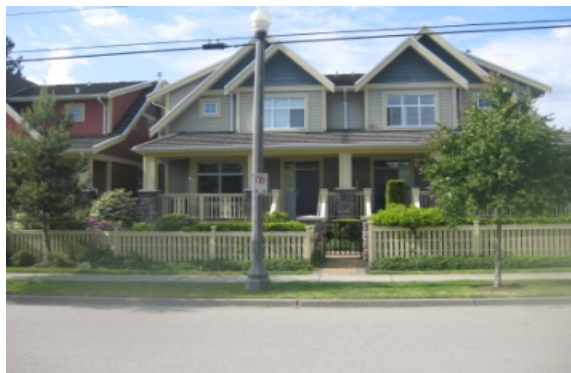
© Darrell W. Kean and Associates Consulting Ltd. 2012. Reproduced with Permission
