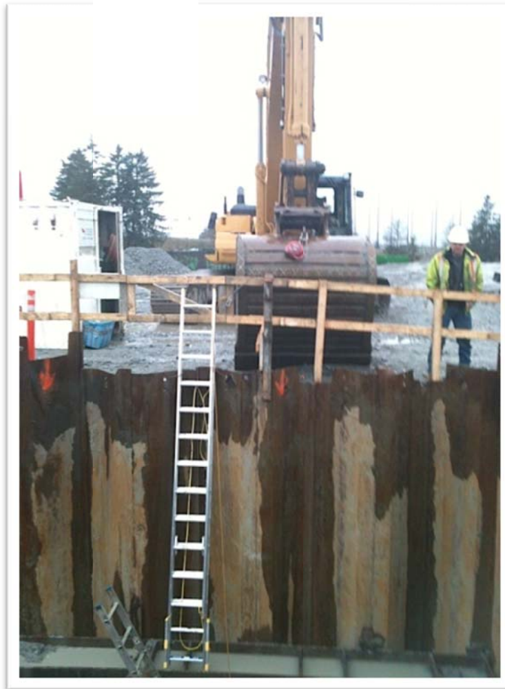
Figure 3.5: Cofferdam (Excavation)
