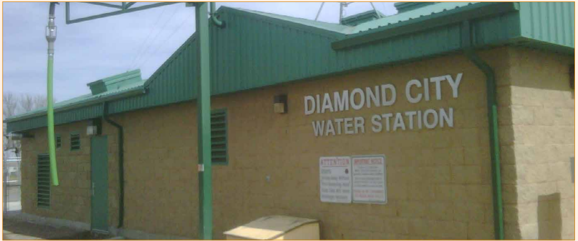
Lethbridge County, Diamond City Water Station
