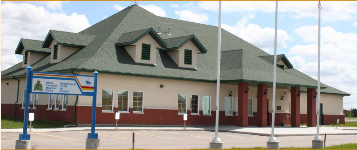
Town of Beaumont, RCMP Building
