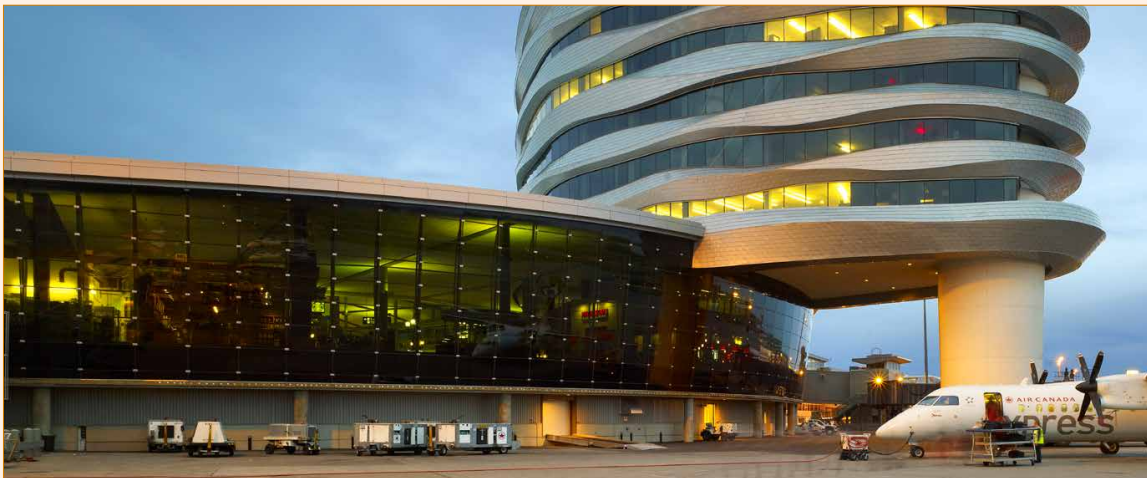
Edmonton International Airport, Control Office Tower
