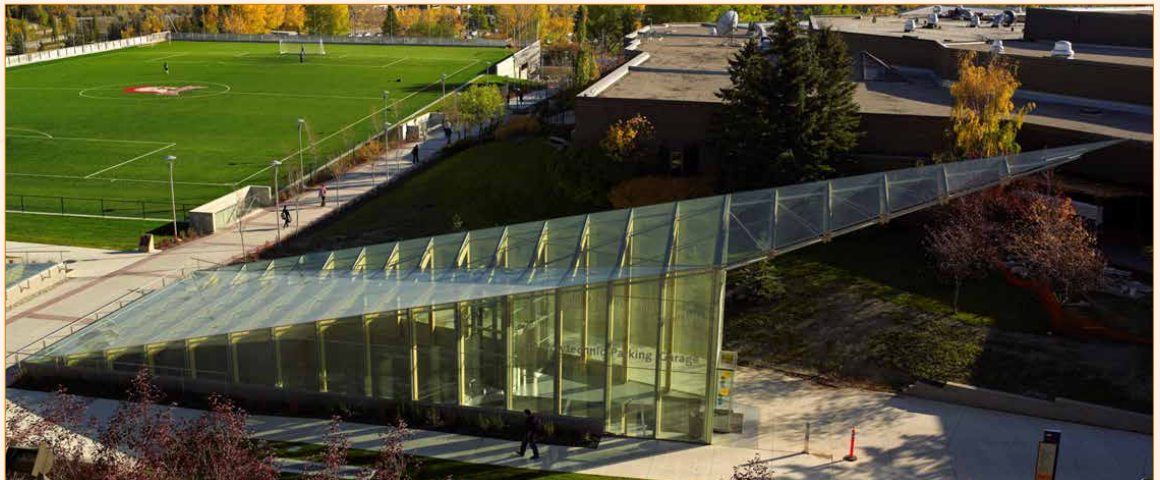
SAIT, Underground Parkade Entrance
