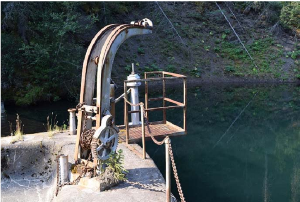
Photo 4 – Part of the existing York Creek diversion system
