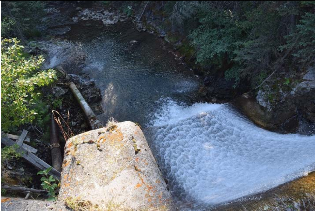
Photo 3 – Drop Structure and Water Release From Dam
