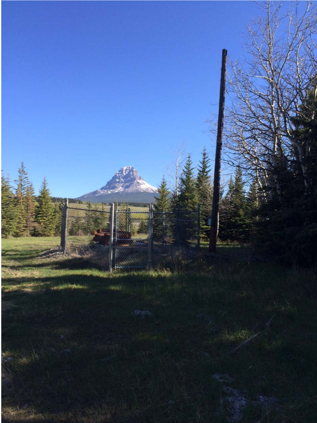
Photo 2 – Part of the Devon Water Intake System on the Crowsnest River
