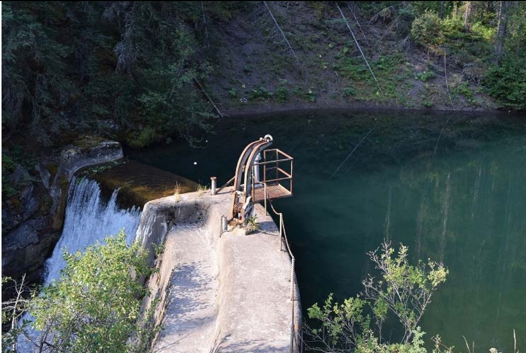
Photo 1 – Dam Structure on York Creek
