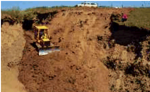
Crawler tractor forming a firm bed for a pipe drop structure.
