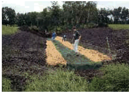
Installing erosion control matting to create a lined channel.
