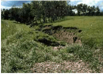
An eroded gully.
