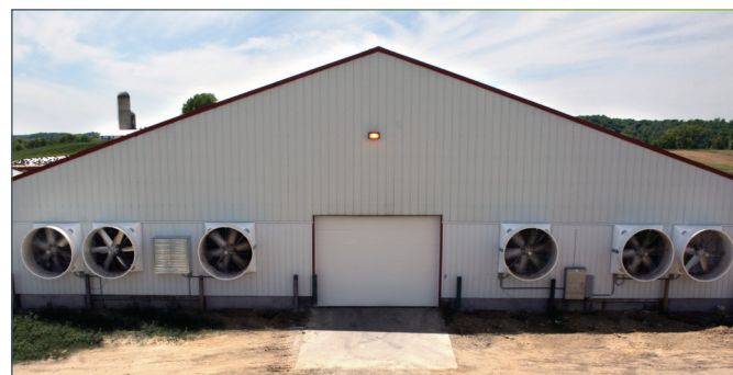
Figure 3. Mechanical Ventilation on Livestock Barn Source: www.jdmfg.com .
