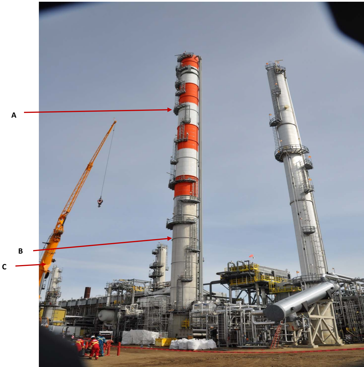
Figure 4. PV-403 (A) was the fractionation vessel where the incident took place. The manway into the confined space was located at (B), and (C) was the crane used to raise and lower the manbasket.
