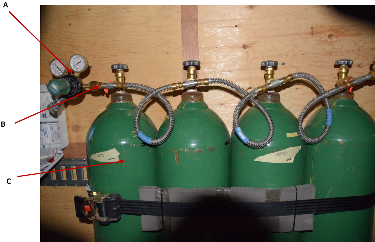
Figure 1. (A) The supplied air cascade system included a first stage regulator, which reduced the cylinder pressure of 2250 psi down to an operating pressure which varied depending on the workers' regulators and masks. The manifold (B) linked all of the cylinders together and equalized the cylinders to one pressure. Each of the cylinders, (C) when filled to operating capacity, contained 300 ft 3 of air at 2250 psi. This was the system that provided air to the workers including the tower mechanic.
