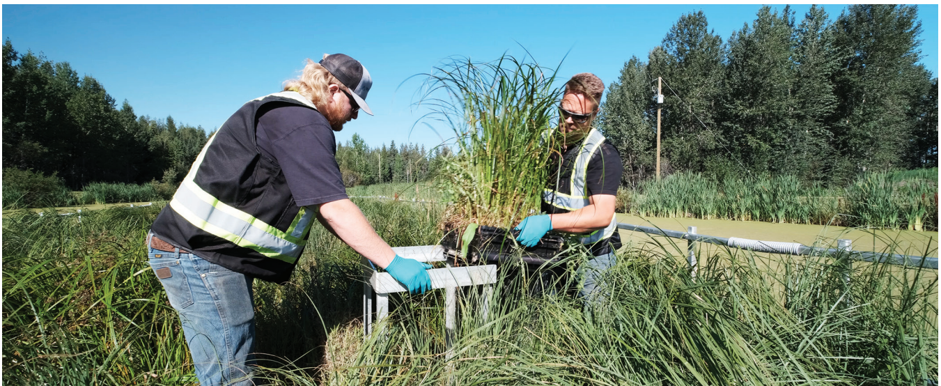
Constructing the Floating Wetlands: Andy Kwirant (left) and Blair Myrfield (right)
