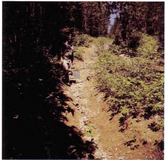
Figure 50. Trails oriented straight up and down slopes can result in damage and gullying even on relatively erosion resistant soils.
