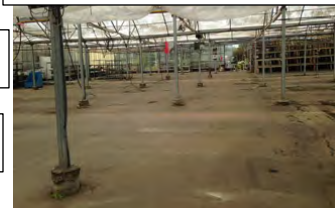
Flood floors at U of S Greenhouses
