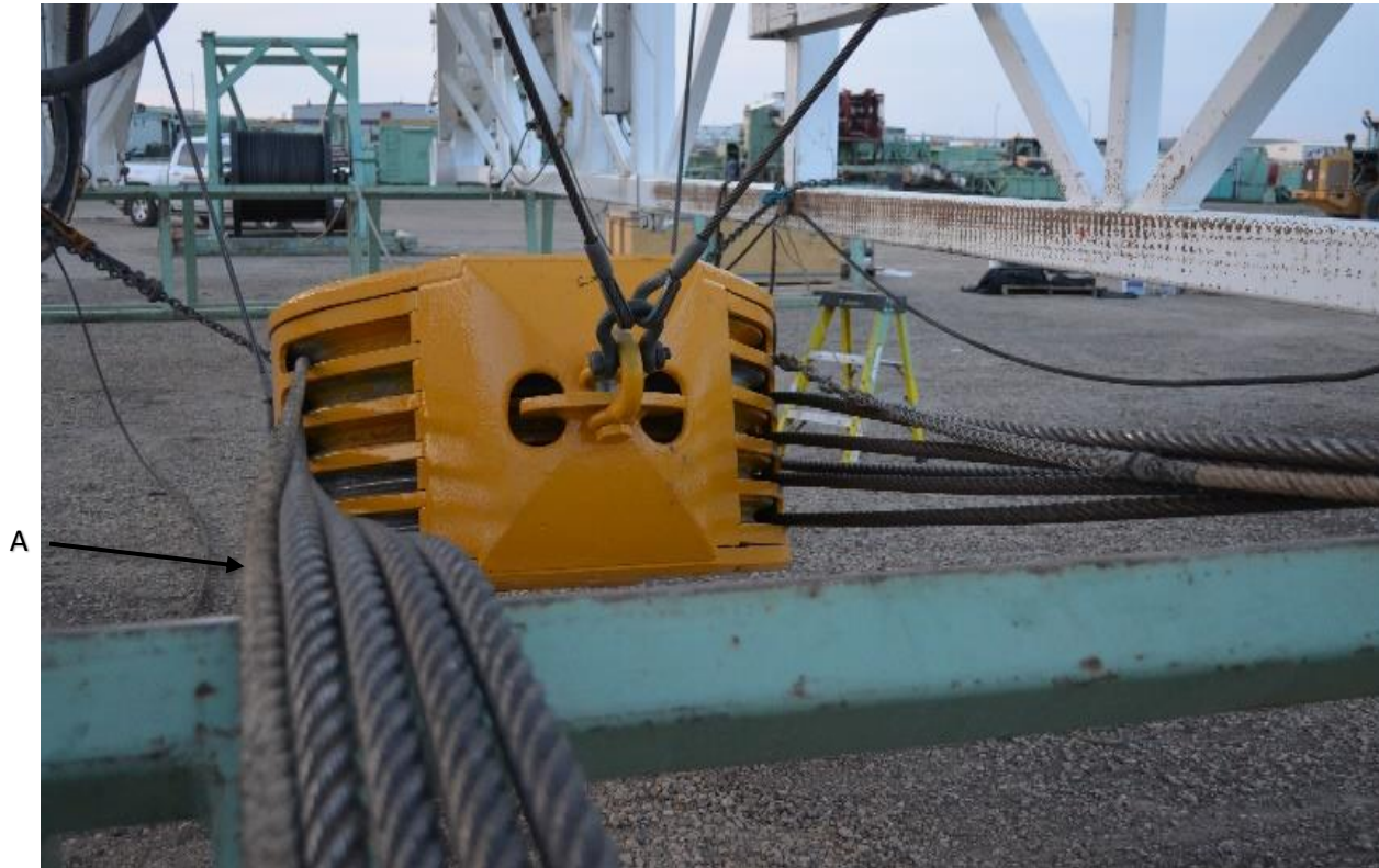
Figure 3. The wire rope drill line that was being threaded or reeved through the travelling block and crown at the time of the incident.
