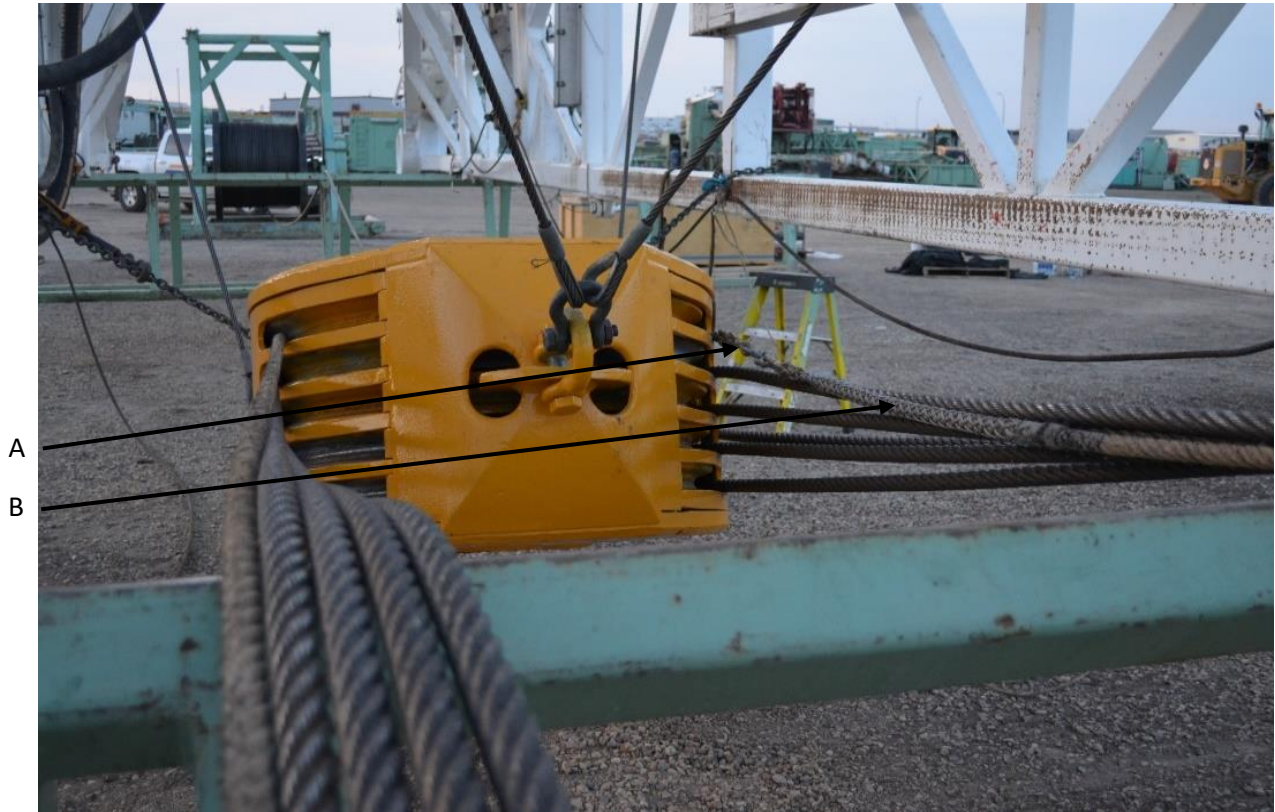
Figure 4. The snake and the pulling rope were attached to the wire rope drill line and were being pulled through the travelling block when the incident occurred. The snake and pulling rope were used to install new cable by using old existing cable to pull the line.
