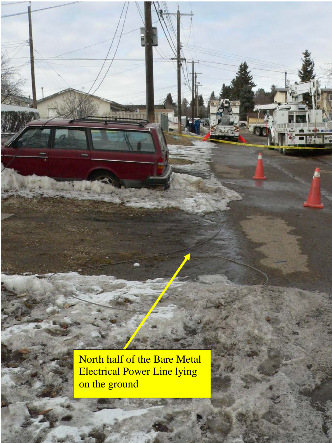
Photograph #11 Shows the severed end of the Power Line between the front of the Radial Arm Digger Truck and the second pole in the alley going north. This line ended up on the ground after being severed.
