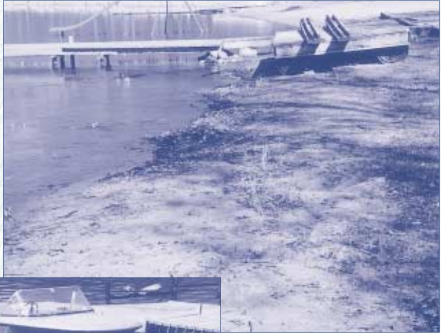
Damaged shoreline – right. All vegetation has been removed and sand has been brought in, creating an unappealing, very sterile shoreline.
