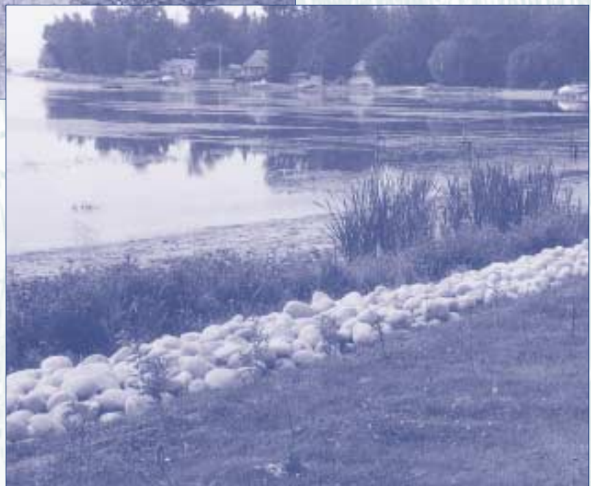
Erosion protection – right, using riprap, aquatic and terrestrial vegetation. All the components will work together to “protect” the bank. The aquatic plants will dampen wave action. The riprap will armour the vulnerable bank, keeping the waves from carrying away soil. The roots of the shrubs behind the bank will also help to hold the soil on the bank in place.
