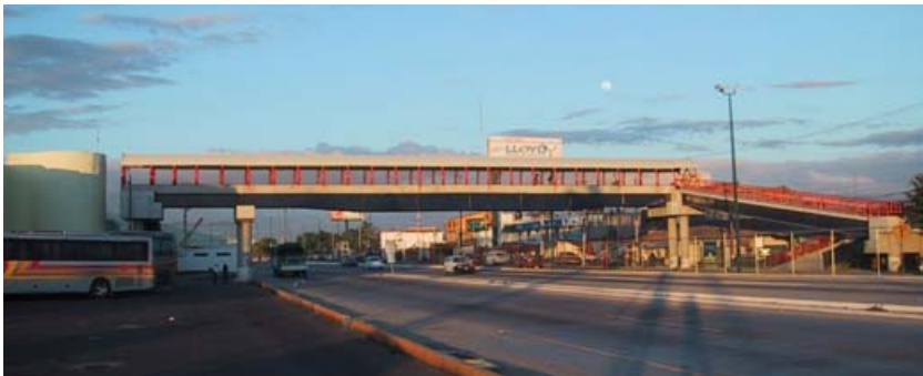
Pedestrian Bridge at Puerto Vallarta, Mexico airport
