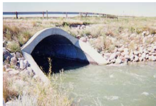
BF 75069 Hwy 36 over Irrigation Canal
