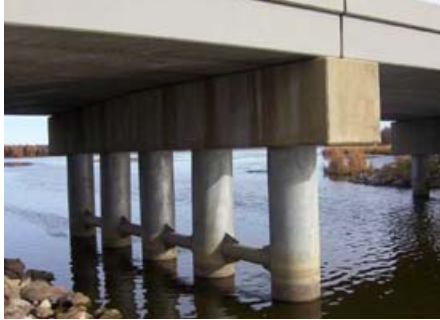
BF 9619 Mink Creek Bridge
