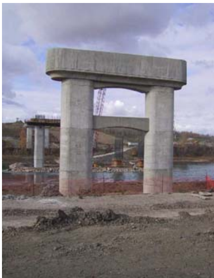
Anthony Henday Drive Over North Saskatchewan River, Edmonton
