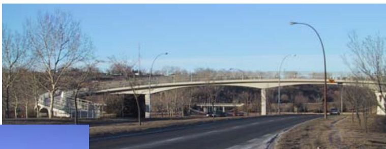
Pedestrian Bridge across Memorial Drive, Calgary (above)
