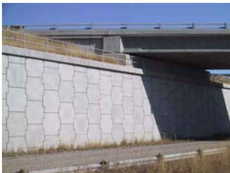
BF 77260 CPR Overpass at Aldersyde
