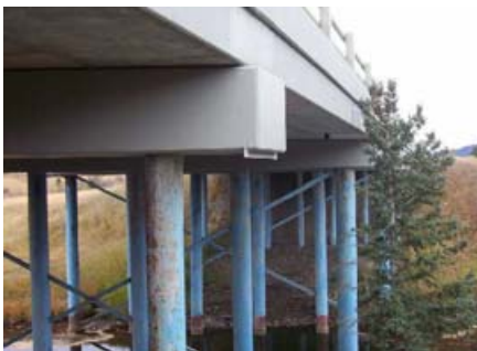
BF 77460 Shunda Creek Bridge
