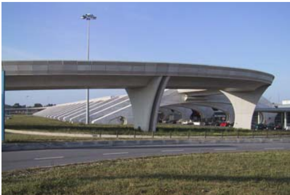
Bridge at airport in Porto, Portugal
