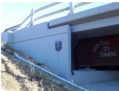
BF 73810E Athabasca River Bridge At Whitecourt
