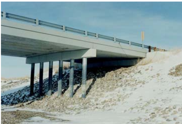
BF 80454 Irrigation Canal near Magrath
