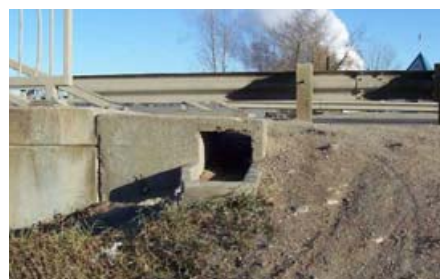
BF 73809E McLeod River Bridge At Whitecourt
