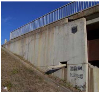
BF 73809E McLeod River Bridge
