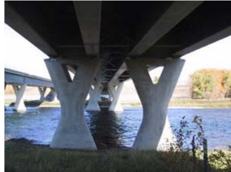
BF 81802 Bow River Bridges, Deerfoot Trail Extension
