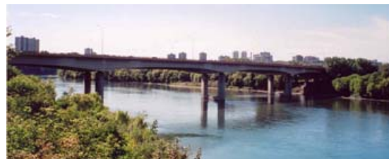
James MacDonald Bridge across North Saskatchewan River, Edmonton
