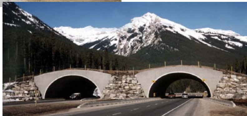
Animal Overpass Structure near Banff (below)
