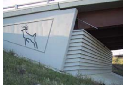
BF 75420E Hwy 2/11 Grade Separation At Red Deer
