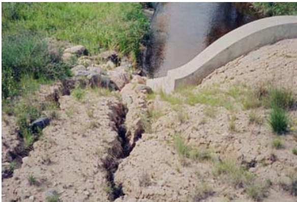
Headslope Erosion
