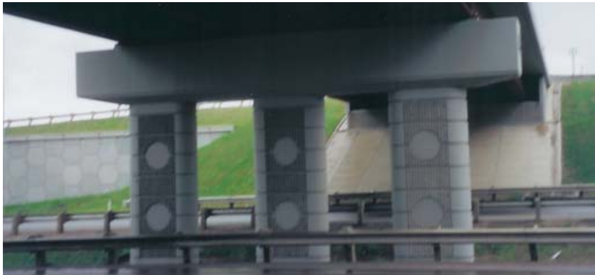
BF 78154 King Street Over Hwy 63 G/S At Fort McMurray
