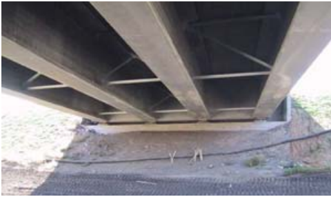
BF 81802 Bow River Bridge Deerfoot Extension
