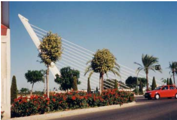
Alamillo Bridge, Seville, Spain (1992) (For description, see Pollalis, 1999)
