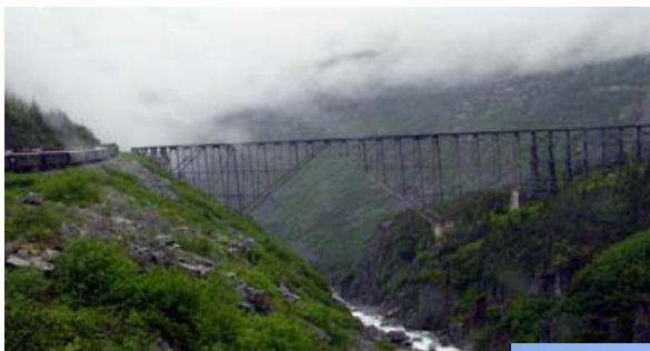
White Pass and Yukon Route Heritage Railroad Bridge, Alaska (above)
