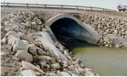
BF 75069 Hwy 36 over Irrigation Canal
