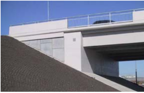
MacKenzie Blvd Over Deerfoot Trail
