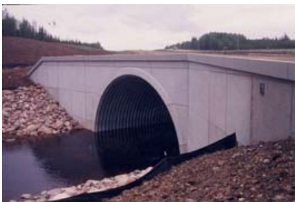
BF 73920E Two Creek Culvert on Hwy 43
