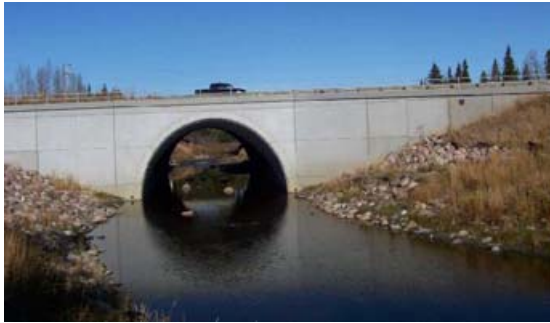
BF 73920E Two Creeks Culvert on Hwy 43
