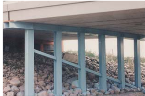
BF 1604 Local Road over Waskatenau Creek
