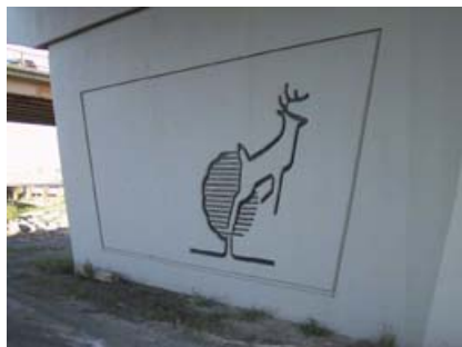
BF 75420E Hwy 2/11 Grade Separation At Red Deer
