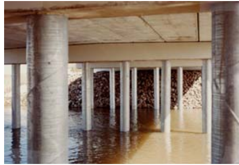
BF 80445 St Mary Canal Bridge NE of Spring Coulee
