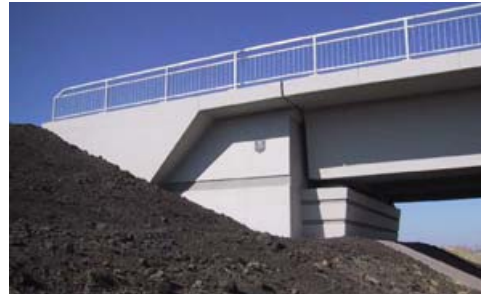
BF 82011 196 th Avenue Over Deerfoot Trail
