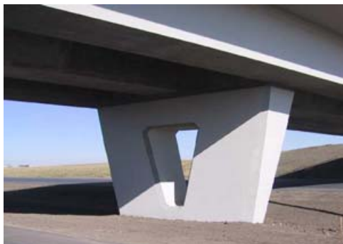
BF 82011 196 th Avenue Over Deerfoot Trail
