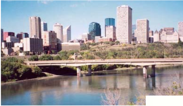
James MacDonald Bridge, Edmonton (above)
