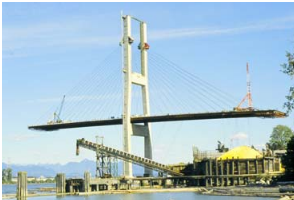
Alex Fraser Bridge across the Fraser River in Vancouver, during construction
