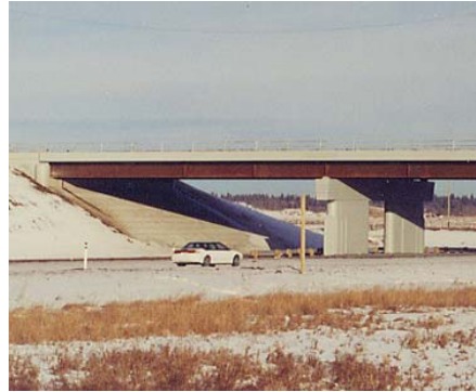
BF 70481 MacKenzie Road over Hwy 2
