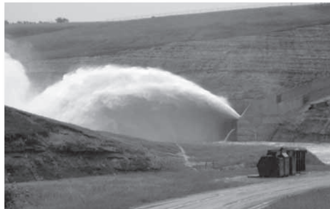
The photos above show the outflow from the St. Mary Dam.
