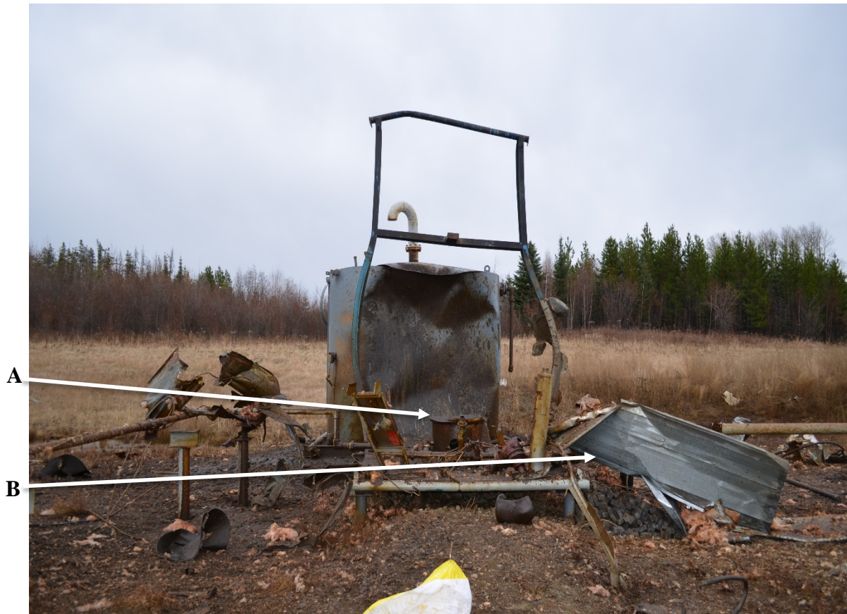
Figure 4. The location of the separator building and remnants of its frame and the vessel were located in various pieces approximately 1000 metres (m) from the base. A manufacturer's identification placard from the vessel stated that Canadian Equipment Sales & Services Co. Ltd. manufactured the vessel on March 20, 1956 (Vessel No. 807) and was rated for a working pressure of 125 psi.
