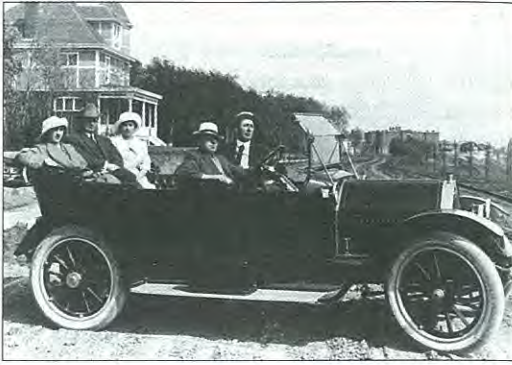
Car on Victoria Avenue, Lessard Residence at left, c. 1913. (GAINA-1328-64562)
