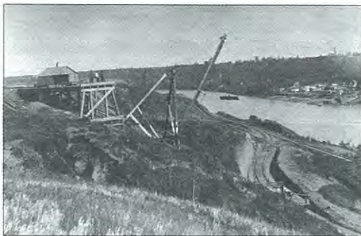
The High Level Bridge under construction c. 1910. (CEA EA-13-1)
