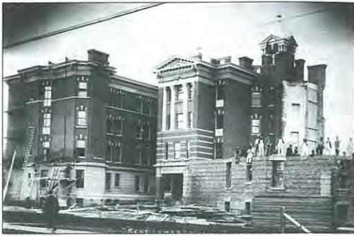
The Lemarchand Mansion under construction c. 1910-1911. (PAA B4224)
