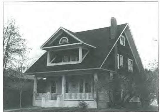
The Ward Residence, 1993. (ACD)
