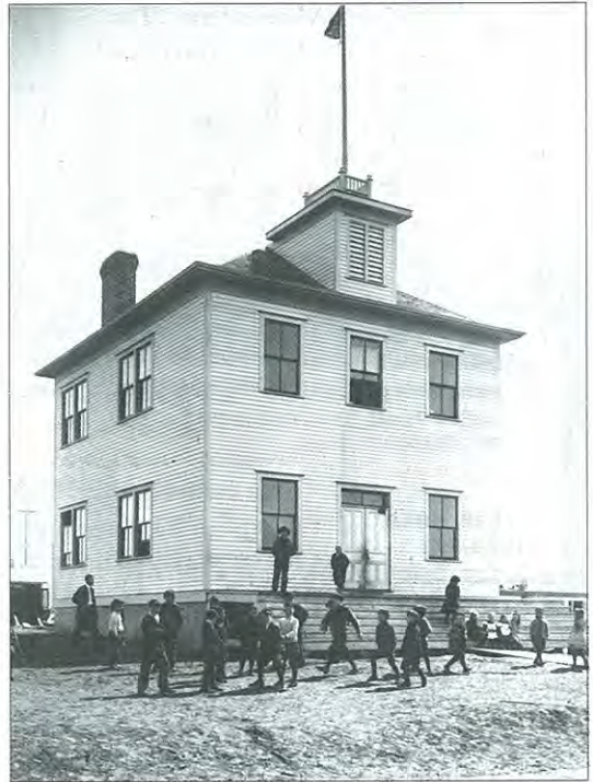
Highlands Cottage School, 1914. (GAI NC-6-760)
