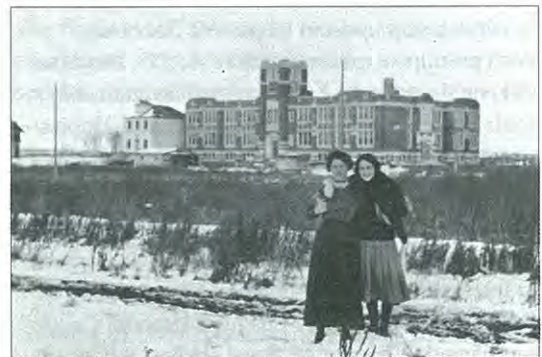
Highlands School, before 1922. (ESBA)
