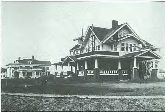
Ada Boulevard houses under construction, 1913. (GAI NA-1328-1136)
