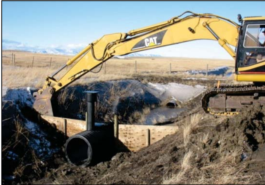
Figure 2.14. Installation of plywood-reinforced berm and flume at Station 17.
